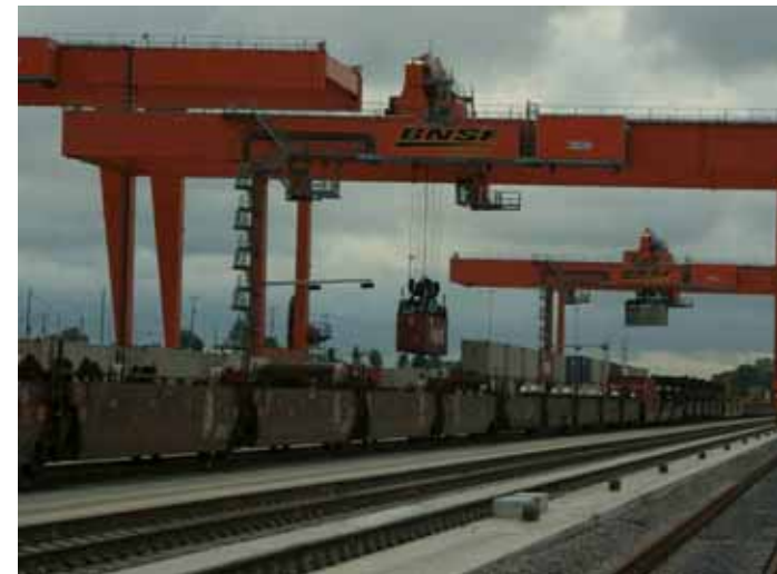
Wide-span Cranes in Memphis
